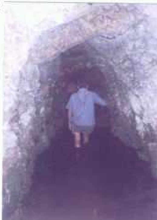
The inside view of an old adit in quartzite. Location- Chongbong
